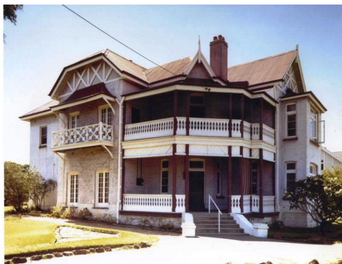
The residence Mozaphir was designed for J.G. Bolton in 1892. Located at the north-west corner of Irvine Street and the Esplanade in Peppermint Grove, it was later owned by the Burt family. It has been demolished. (courtesy Julian Burt).
