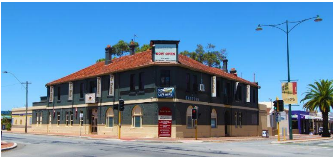
Freemasons Hotel Helena Vale (Midland) opened in 1897. Encircling verandahs have been removed. (Google Maps 2014).
